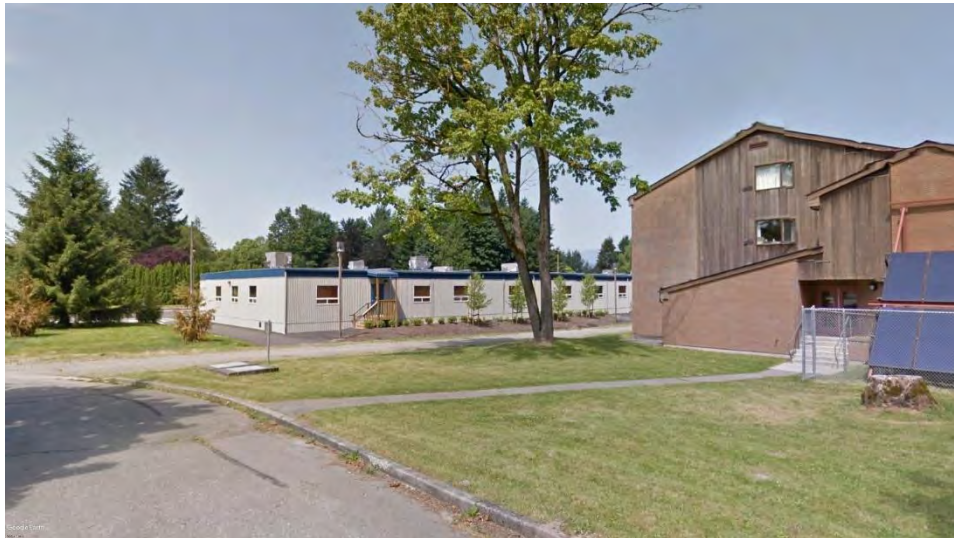
View of Student Residence building and classroom block
