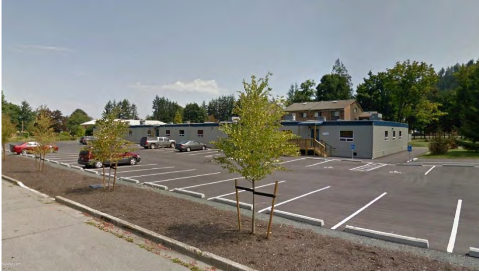
View of classroom block from parking area
